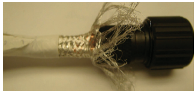
Figure 41: Brushing the braid
