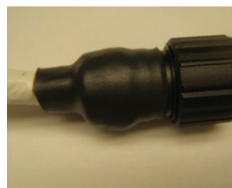
Figure 49: Shrinking tubing on plug
