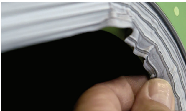
Figure 26: Wrapping the tape around a curve
