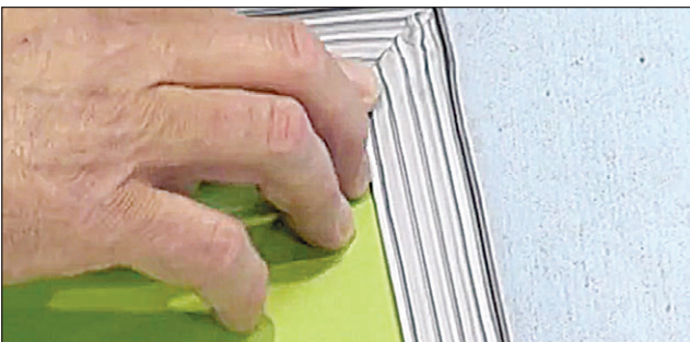
Figure 32: Continuous seal around the top of the corner
