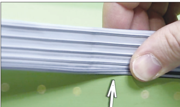
Figure 21: Positioning tape on panel edge
