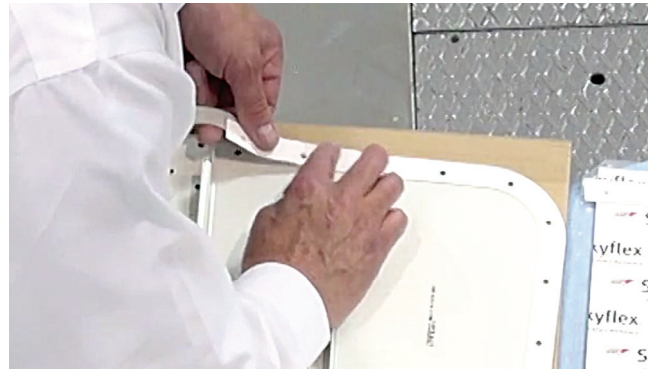
Figure 4: Applying pressure to the gasket
