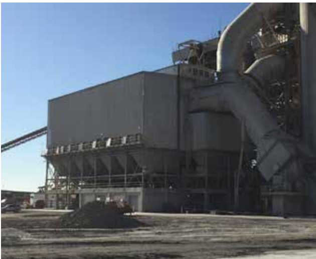
Figure 1. The reverse air baghouse cleans at a rate of 1.513 million acm/hour.
