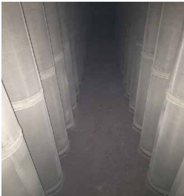
Figure 6. After 8 months in operation, the GORE LOW DRAG filter bags compartment is dust free.
