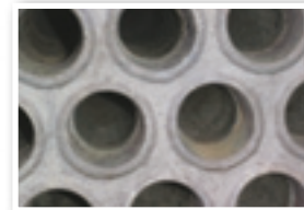
Sulfur Recovery Unit After Cleaning with NitroLance
