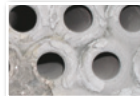
Sulfur Recovery Unit Before Cleaning with NitroLance
