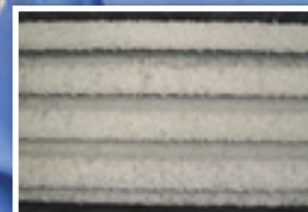
Economizer Enhanced Fin Tubes O.D. Before Cleaning with NitroLance
