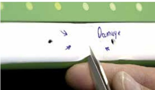
Figure 9: Slitting the damaged section
