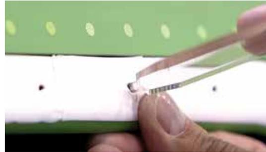
Figure 14: Punching a fastener opening
