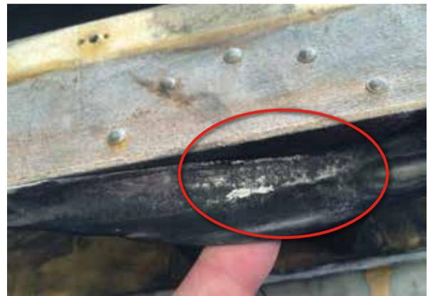
Figure 6: Repair required for delaminated tape separated from the panel.
