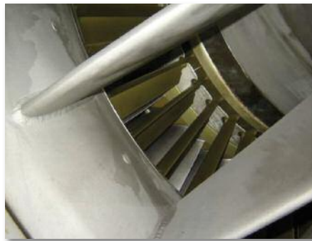
Figure 6. Boroscope picture of compressor section of LM6000 fitted with Gore filter, after 10600 hours, showing totally clean blades
