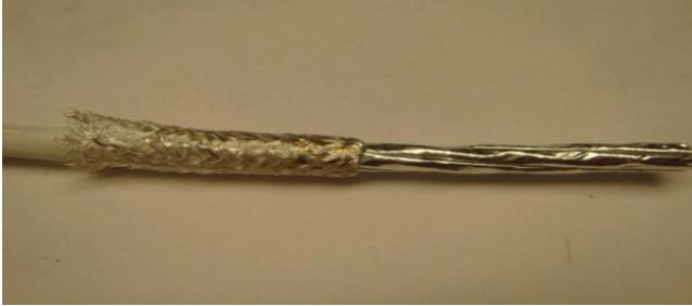
Figure 16: Exposing the foil
