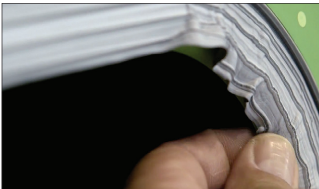
Figure 26: Wrapping the tape around a curve
