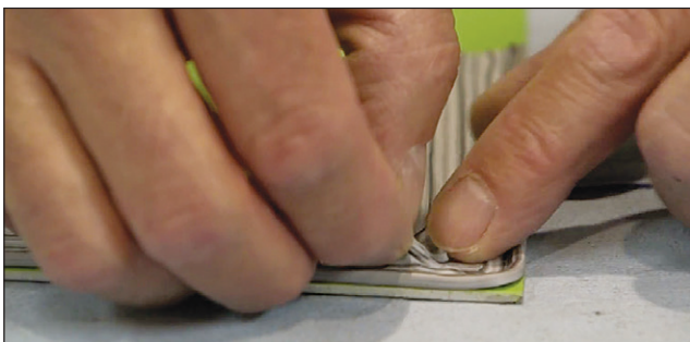
Figure 31: Overlapping the tape
