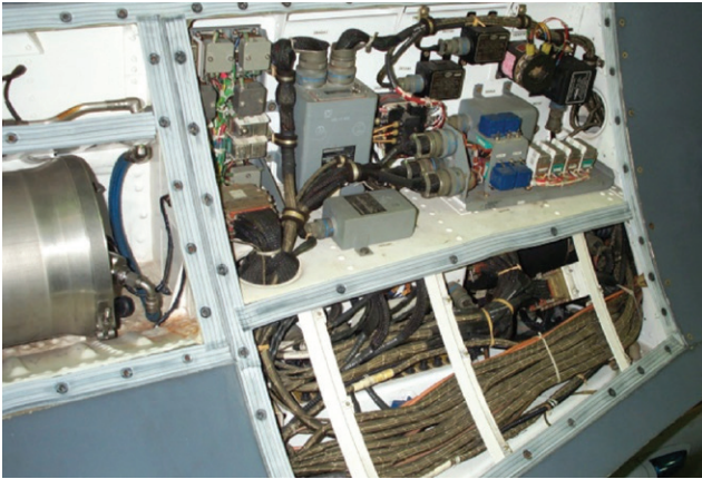
Figure 2: Airframe installation for panel 2406
