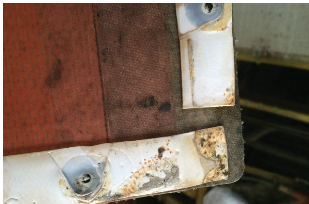
Figure 5: Improper corner overlap and gap between materials
