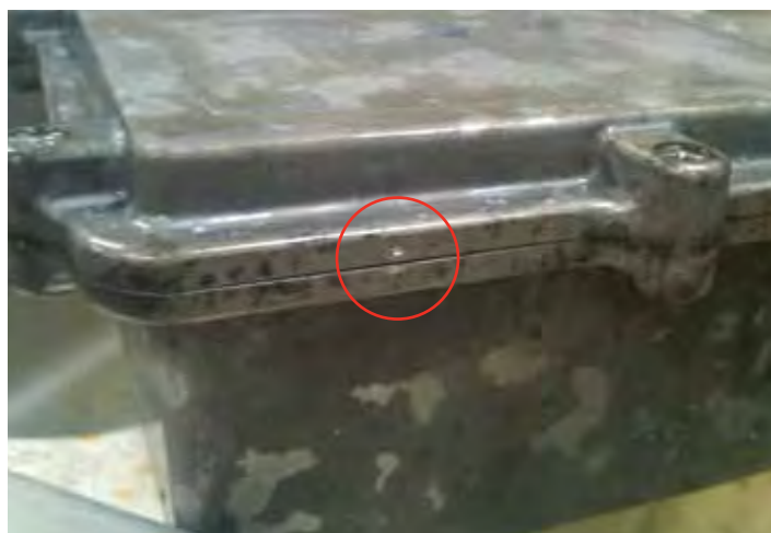
FIGURE 7: ENCLOSURE VISUALLY INSPECTED AFTER THE TESTING
