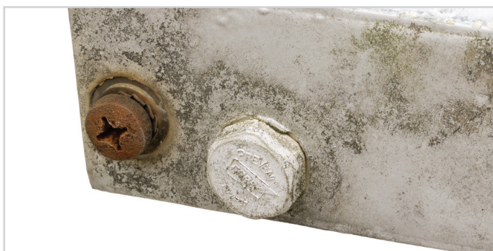
FIGURE 2: SCREW-IN VENT POSITION ON SAMPLE EQUIPMENT
