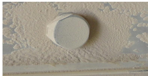
FIGURE 4. Outside of Module After Test.
