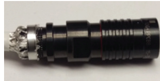
Figure 47: Trimming excess braid on plug
