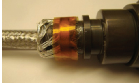
Figure 72: Wrapping Band-It® clamp
