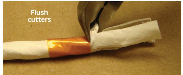
Figure 16: Cutting the two flaps
