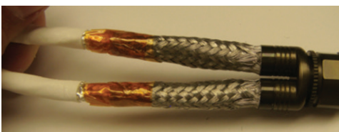
Figure 47: Taping the braid
