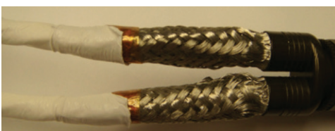
Figure 48: Repositioning the outer jacket
