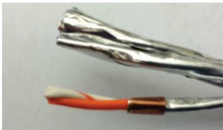
Figure 36: Removing the foil edge
