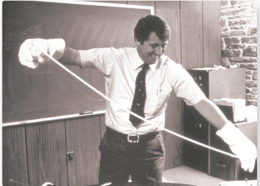
Rapid application of tensile force to heated PTFE changes the polymer's microstructure, as Bob Gore discovered in 1969. Atomic-force microscopy reveals that PTFE's spiraled nodes expand into a network of nodes and fibrils. The network can be as much as 70% air, depending on expansion conditions.
