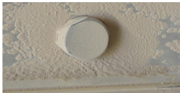
FIGURE 4. Outside of Module After Test.
