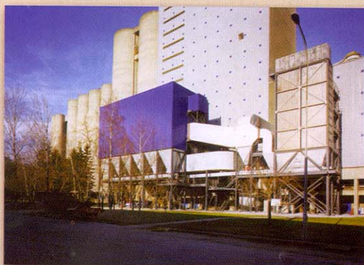
Combined clinker cooler and Lepol kiln dedusting at Ciments d'Origny, Rochefort.
