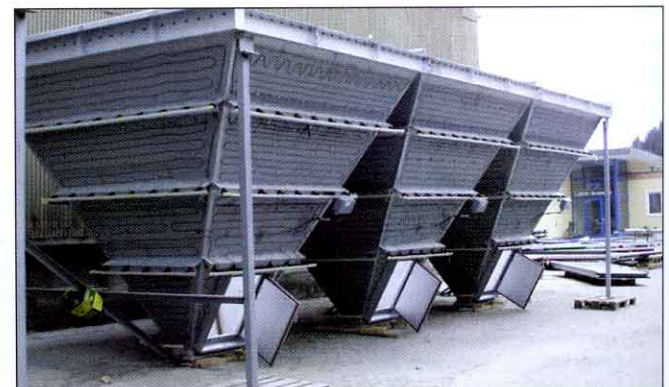
Figure 6: hopper preassembly on site
