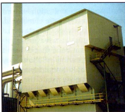
Figure 1. The TGT baghouse at Lafarge Paulding.
